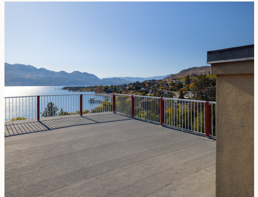
The roof deck
